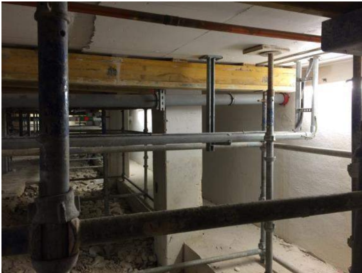
Figure 3: Propping to underside of Level 9 building D1.3
