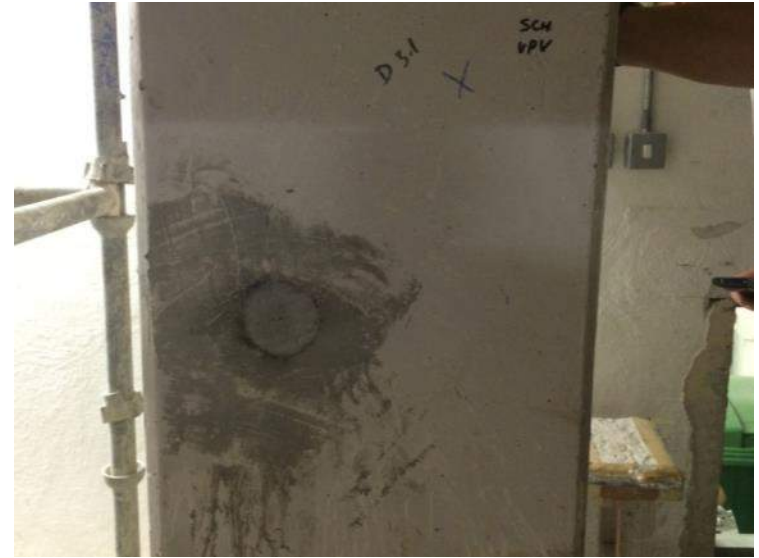
Figure 2: Repaired core
