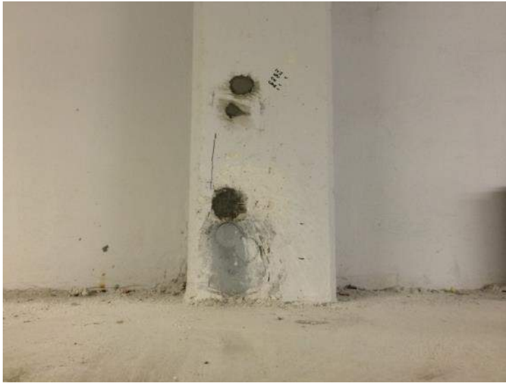
Figure 1: Multiple cores in single column
