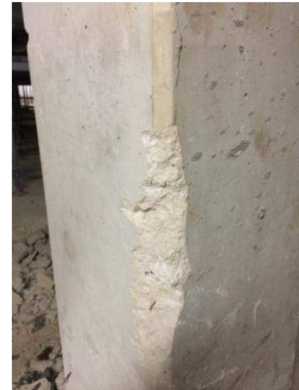
Figure 4: 'White' concrete column (D1.3)
